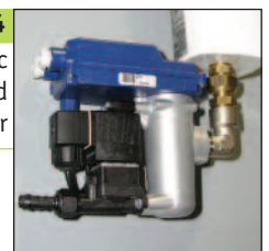
BEKO 12 electronic drain fitted on the filter
